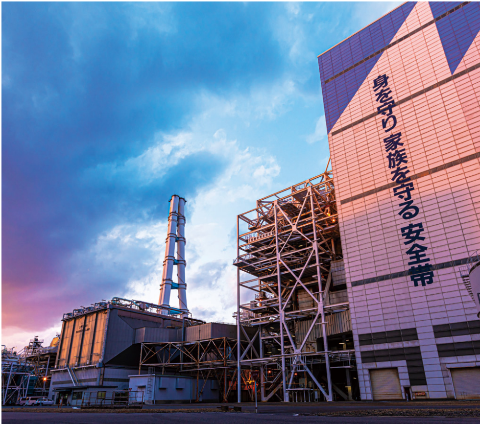
Safety is a top priority at Hekinan Thermal Power Station (Hekinan City, Aichi Prefecture), where ammonia demonstration tests are scheduled to begin in FY2023. Safety belts (fall arrest devices) and other safety equipment are being installed across the facility.
